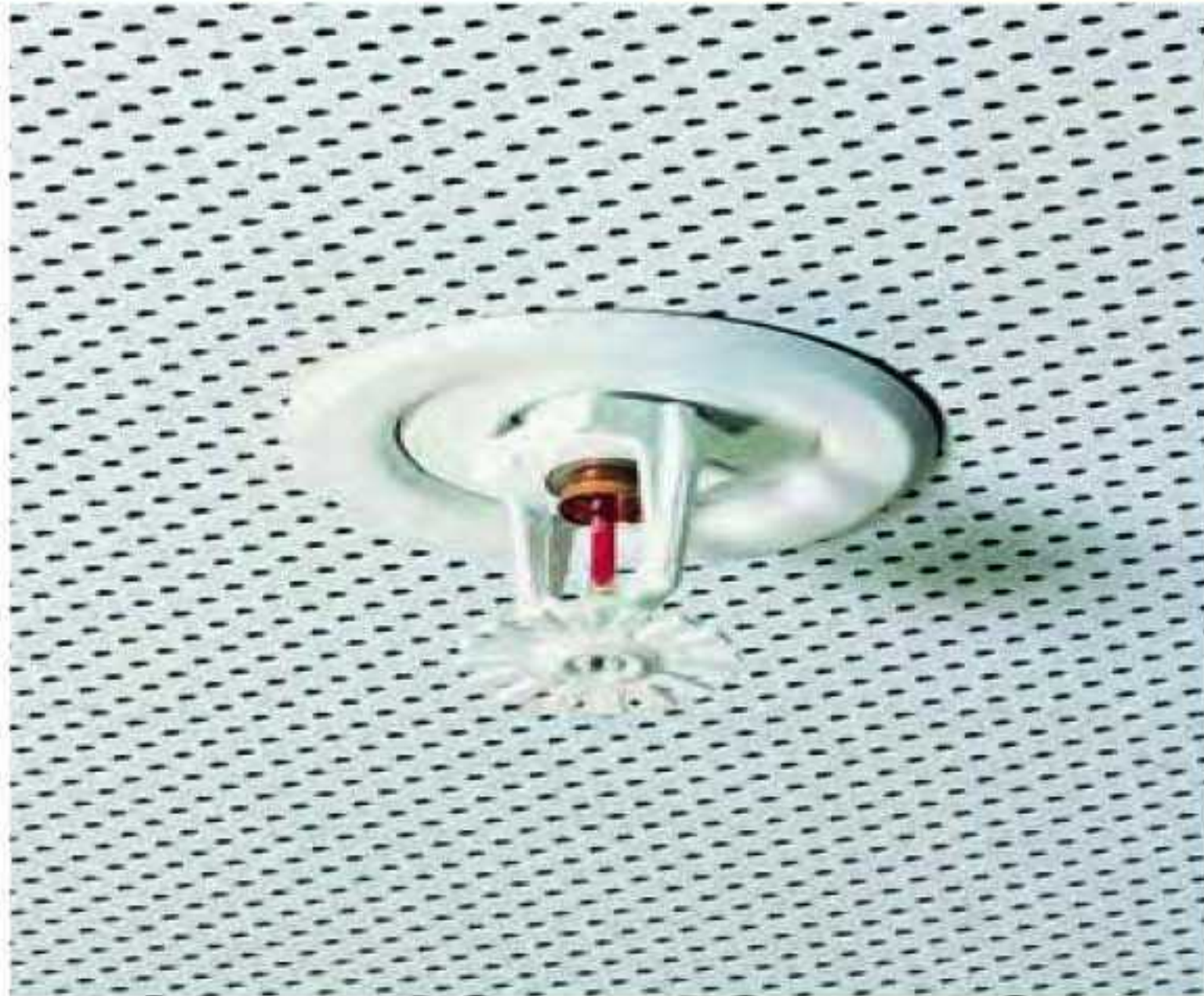
Sprinkler head fitted through circular cut-out
