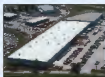
Hunter Douglas Fabrication, Slacksmead (GA), U.S.A.
