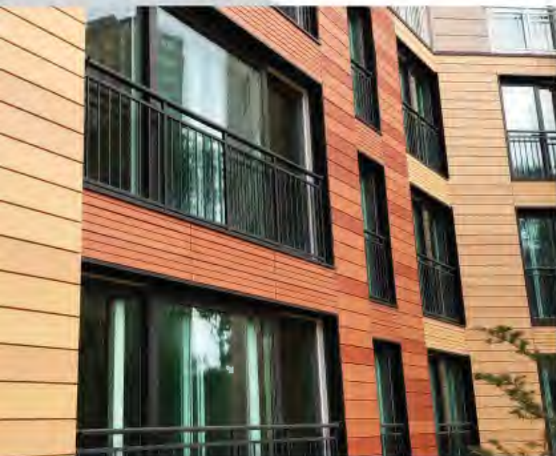
Shindong Raemian Apartments, South Korea NBK Mid 3
