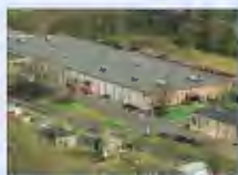
Hunter Douglas Fabrication, Willow Grove (PA), U.S.A.
