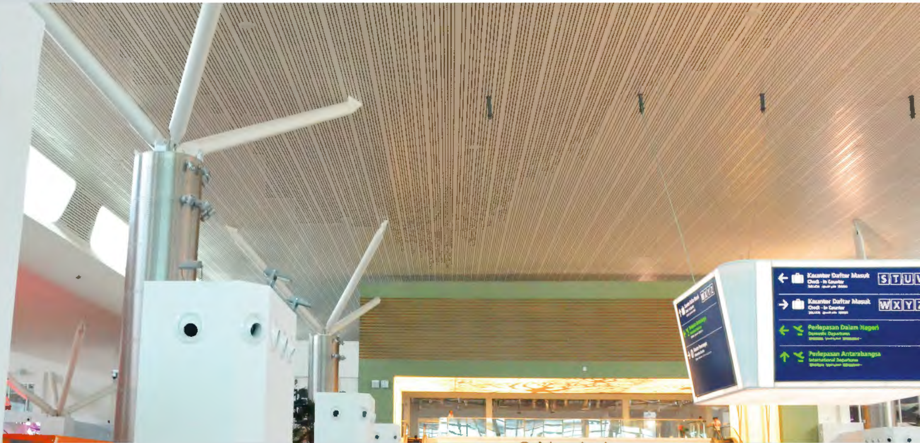
KLIA2 Malaysia Multi B ceiling
