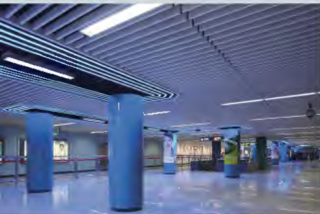
Shanghai Metro Station Line 1 U-Baffle
